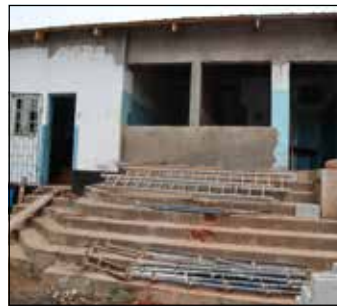
Construction at Zomba Theological University in Malawi.
